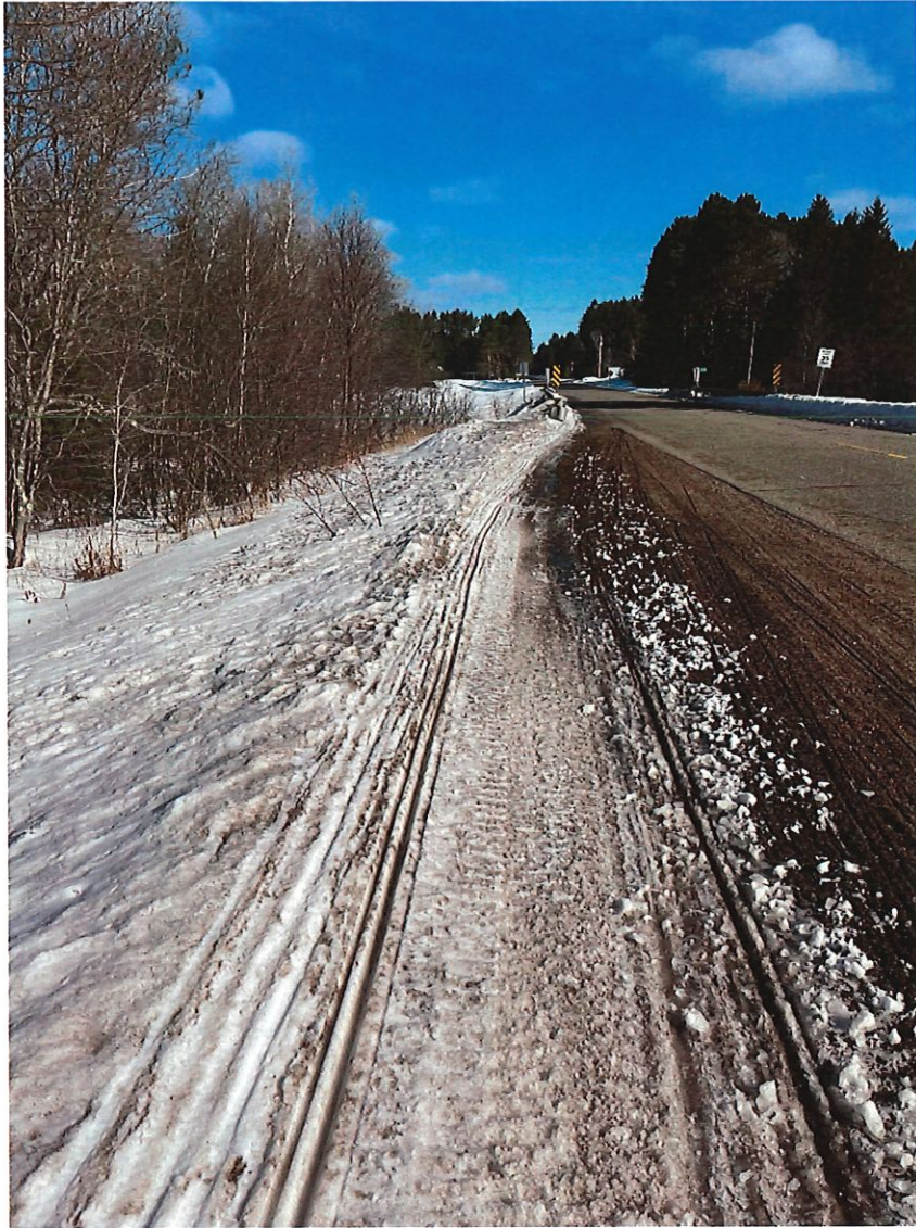
South of Bridge Looing North
