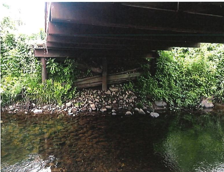
Bridge Substructure and Abutment Looking West
