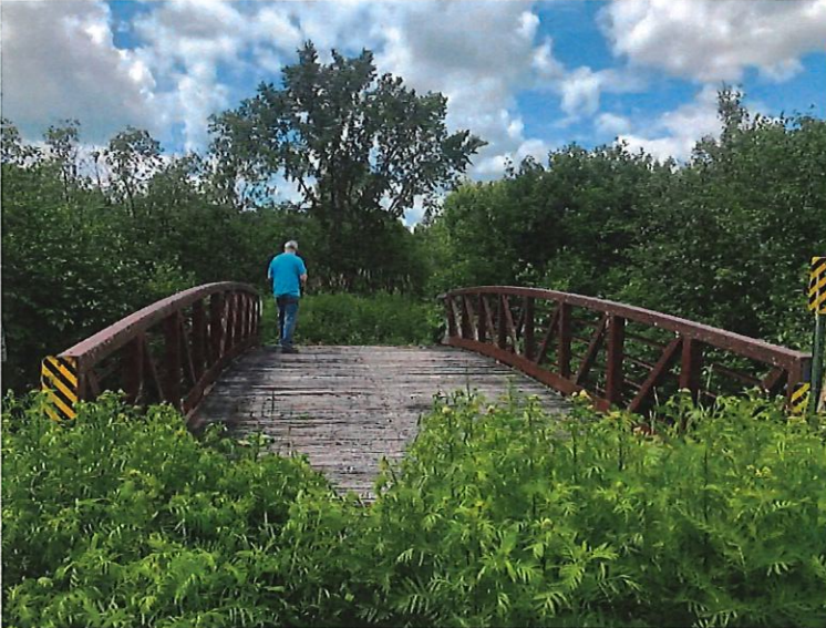
Bridge Deck Looking West
