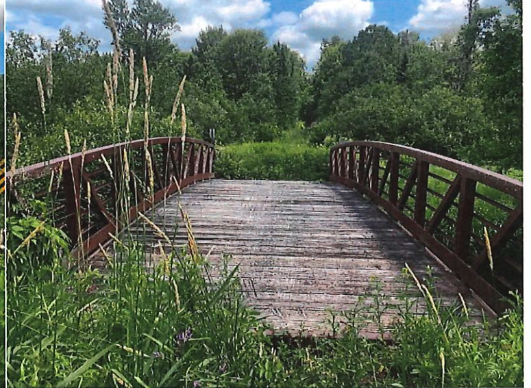
Bridge Deck Looking East
