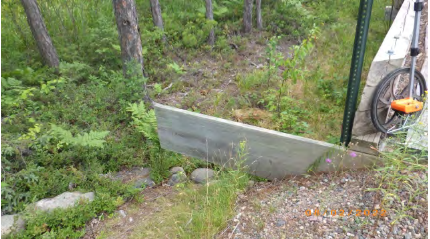
Typical Backing boards for all bridges,
