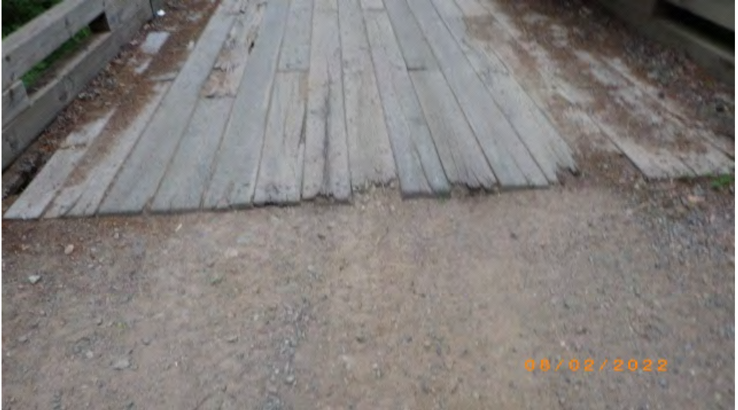
B3- 2inch settlement and CS3 deck boards.
