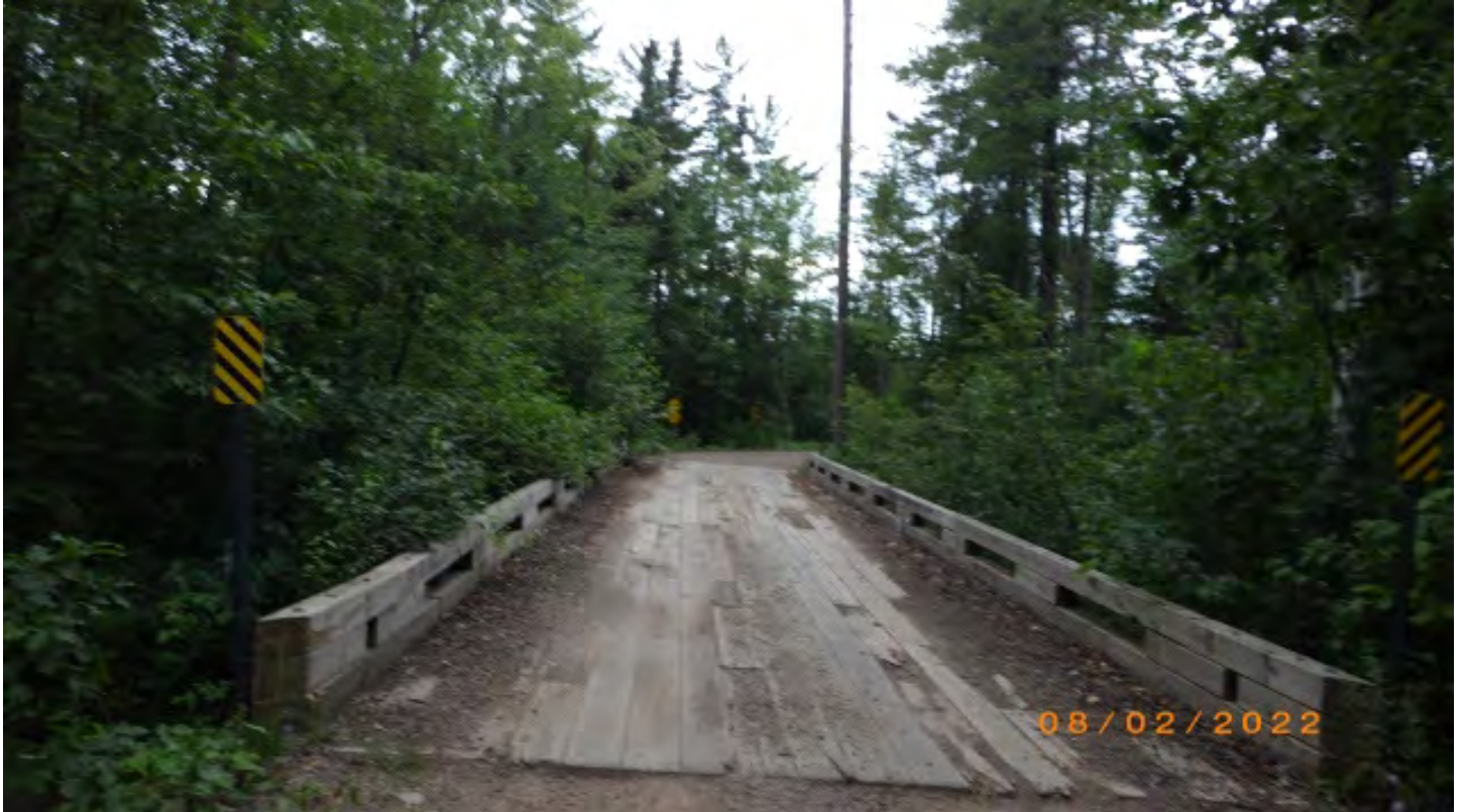
Cut brush typical of all the bridges.
