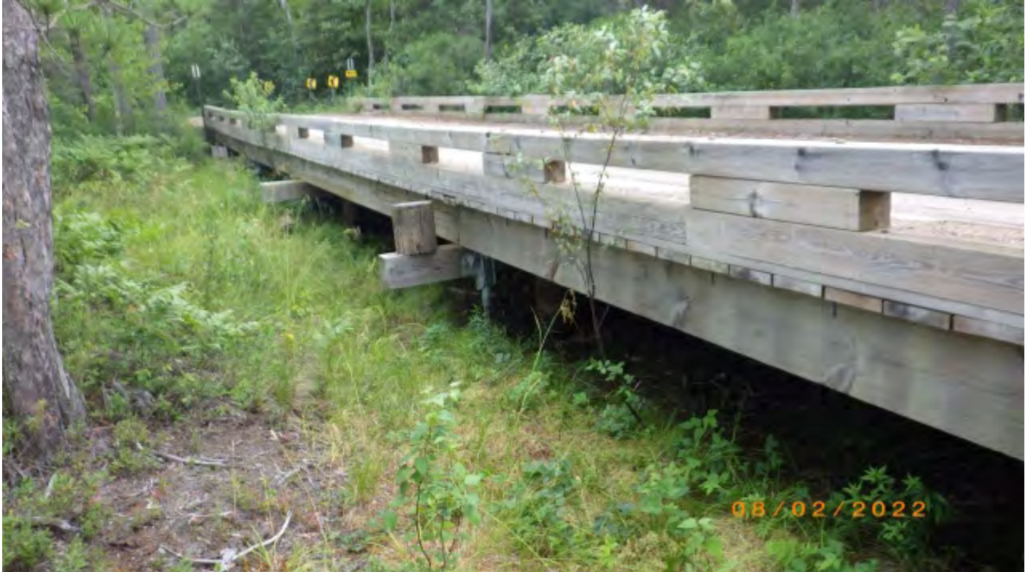
Elevation view of B2, typical of all 4 bridges.
