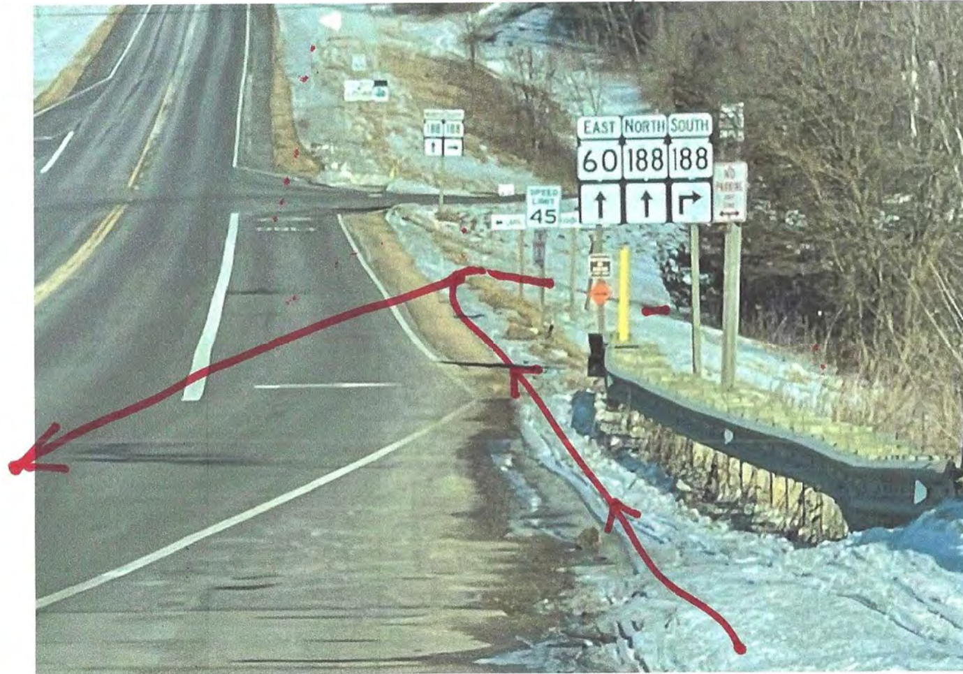
East Side of Bridge
