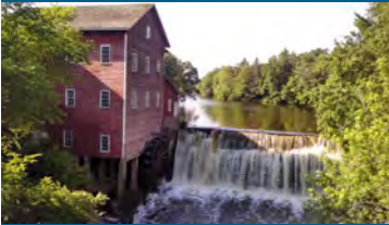
Dells Lake Dam
