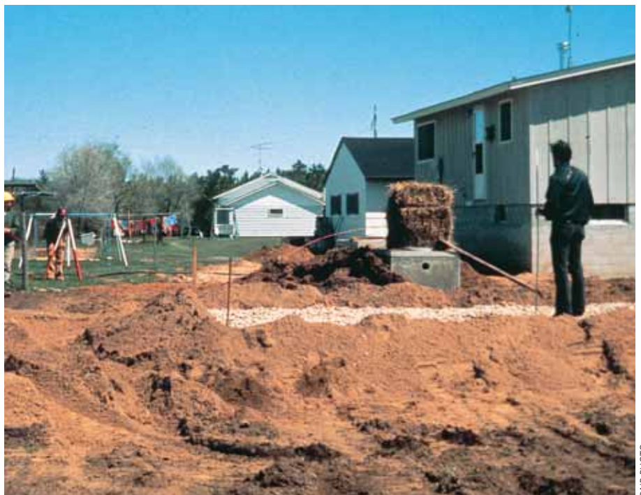
Installing a sewage drainage field.
