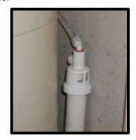
Manufactured air gap for water treatment backwash
