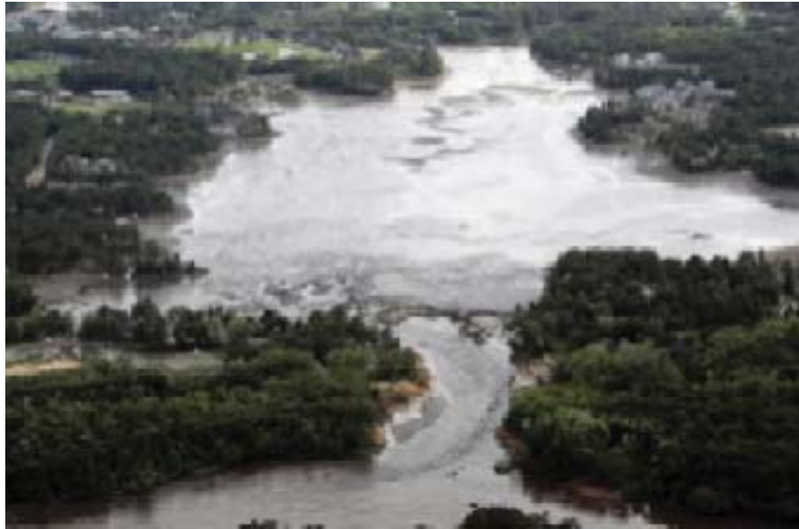
- Breach at Lake Delton, June 12, 2008
