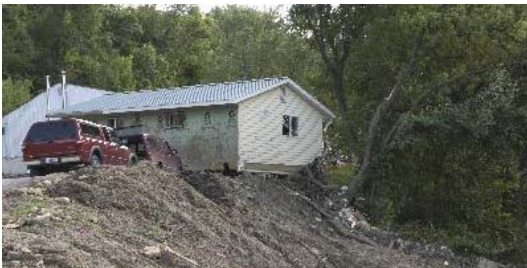
- Flood damaged home, La Crosse, WI 2007
