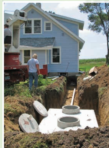
Septic System Installation
