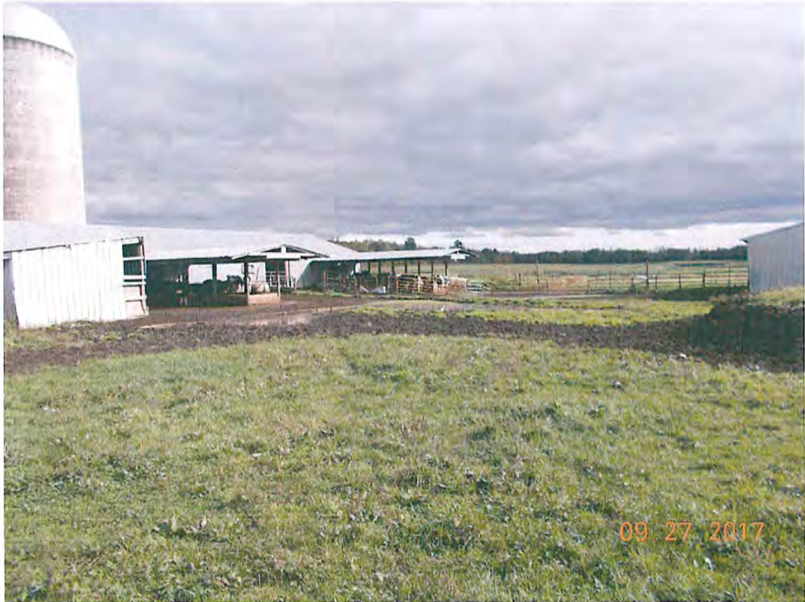
This photograph is taken from Field 8 looking southeast into Fields 7-0 and 7-1. Concentrated feeding is done along the buildings, with runoff travelling down the farm road into the unnamed waterway.
