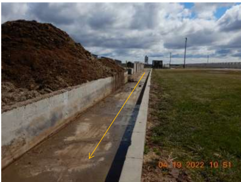
Photo 5. A concrete channel that conveys runoff from the calf hutch area to the manure recirculation basin. The orange arrow represents the flow path of runoff. This photo was taken facing east.
