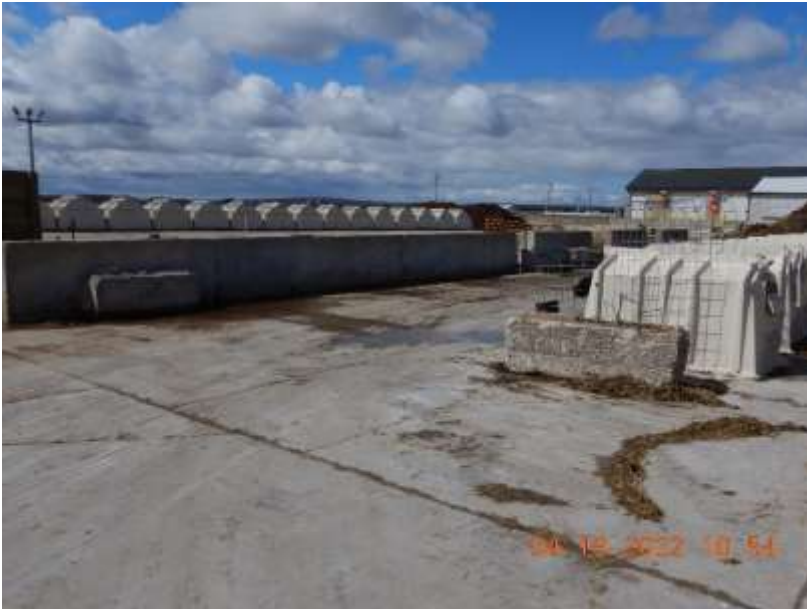
Photo 7. The calf hutch area located east of the sand land. Runoff from this area flows to the southwest corner where it enters a concrete channel that gravity flows to the manure recirculation basin. This photo was taken facing west.
