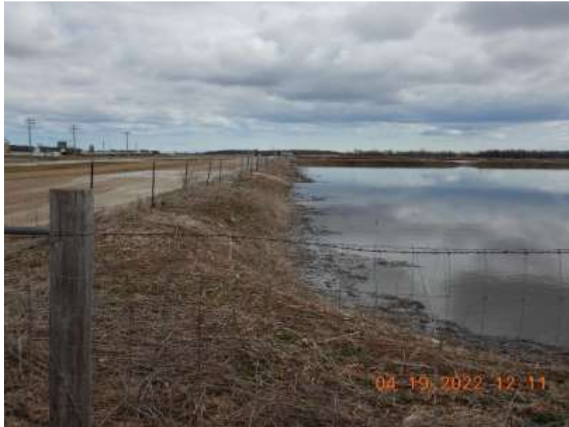
Photo 36. Erosion present adjacent to an agitation pad within WSF 3. Rainwater runoff from the pad caused the erosion.
