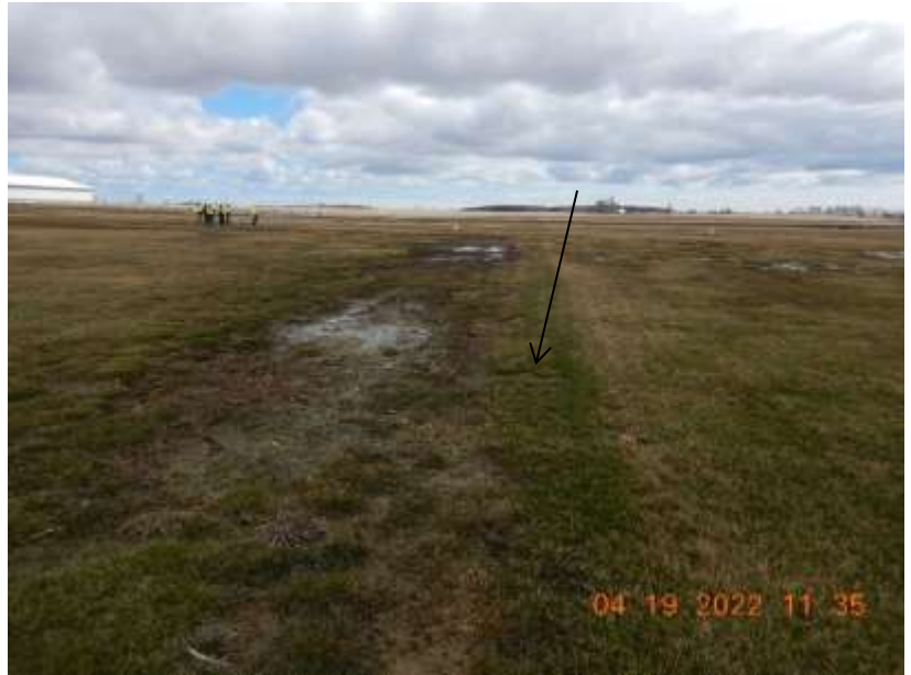
Photo 72. An earthen berm in the middle of the vegetated treatment area. The berm slows the flow of runoff, causing ponding within the treatment area.
