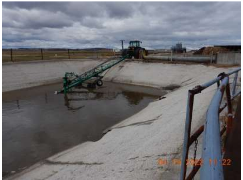
Photo 19. WSF 4, located east of the feed storage area. WSF 4 accepts runoff from the feed storage area. This photo was taken facing south.
