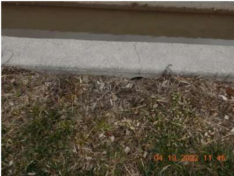
Photo 83. A concentrated flow channel coming from the east side of the concrete spreader bar for the east VTA. This photo was taken facing south.
