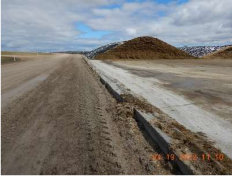
Photo 54. The feed storage area at the Main Site. Haylage and corn silage are stored in piles, covered with plastic. Runoff flows to the southeast corner of the feed pad.
