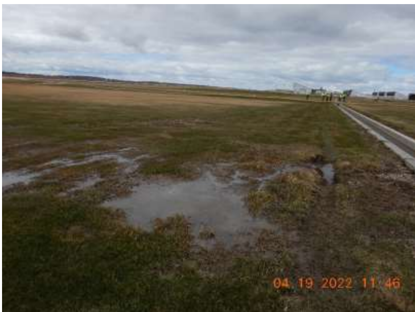
Photo 84. A concentrated flow channel coming from the east side of the concrete spreader bar for the east VTA. This photo was taken facing west.
