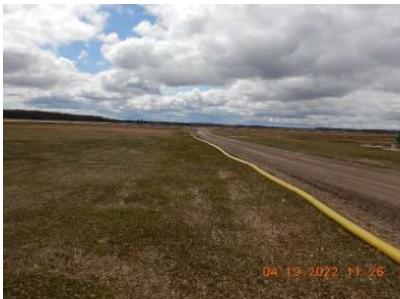
Photo 22. The overland transfer hose that is used to transfer process wastewater from WSF 4 to WSF 3. This photo was taken facing south.
