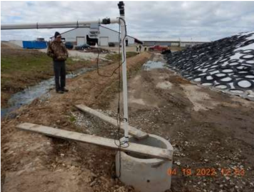
Photo 95. The runoff collection system for the feed storage area at the Heifer Dreams site. The basin is located in the southeast corner of the FSA.
