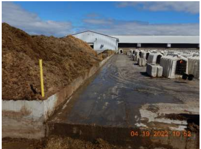
Photo 5. A concrete channel that conveys runoff from the calf hutch area to the manure recirculation basin. The orange arrow represents the flow path of runoff. This photo was taken facing east.
