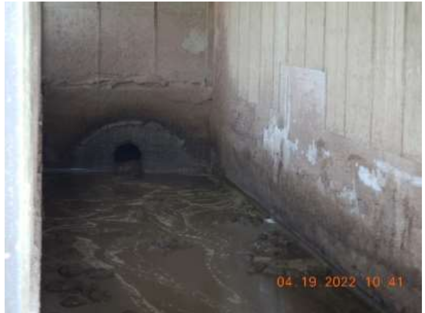
Photo 10. The outlet that discharges manure generated at the Main Site to the north side of the sand lane.
