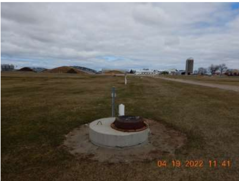
Photo 78. The basin that captures runoff from the concrete swale and pumps the water to either the concrete spreader bar or WSF 4. This photo was taken facing north.
