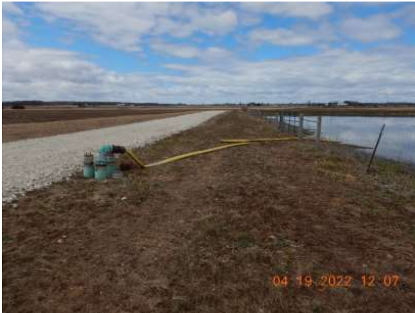
Photo 33. Animal burrowing present near an agitation pad in WSF 3. Gravel and bentonite that was used to fill the hole was dug out.
