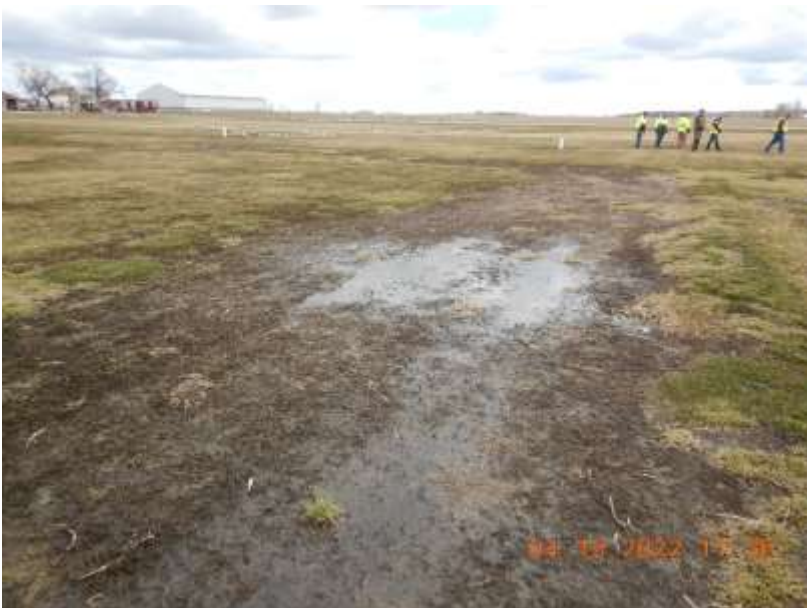
Photo 72. An earthen berm in the middle of the vegetated treatment area. The berm slows the flow of runoff, causing ponding within the treatment area.
