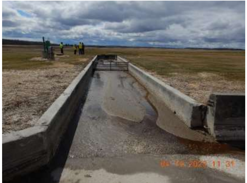
Photo 66. The runoff collection system for the feed storage area at the Main Site. This is located on the southeast corner of the FSA. This photo was taken facing north.
