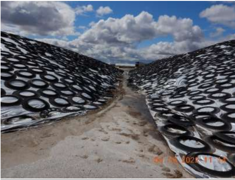
Photo 59. One of two collection inlets associated with the feed storage area. This inlet collects a small percentage of runoff from the feed storage area and transfers the runoff to the east vegetated treatment area.
