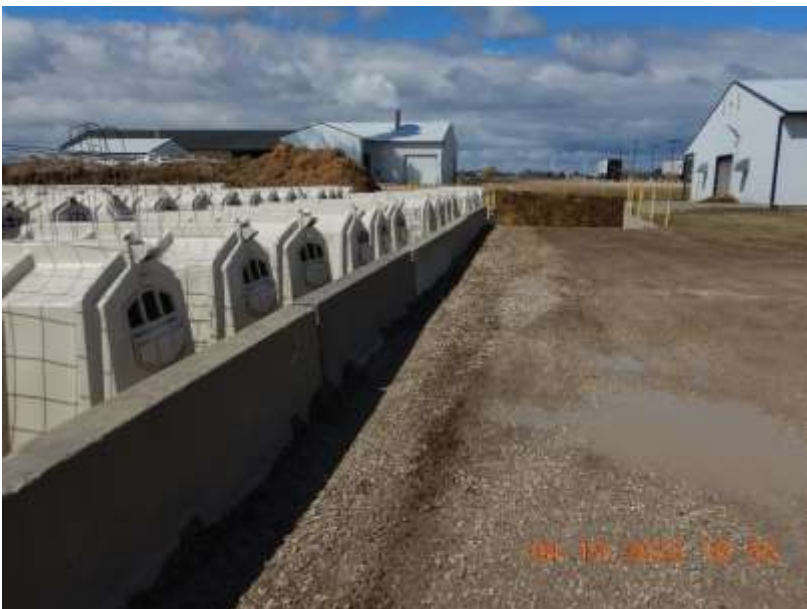
Photo 8. The calf hutch area located east of the sand land. Runoff from this area flows to the southwest corner where it enters a concrete channel that gravity flows to the manure recirculation basin. This photo was taken facing west.
