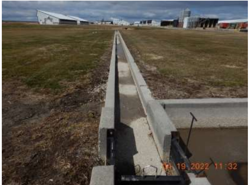
Photo 69. A concentrated flow channel on the east side of the west vegetated treatment area. This photo was taken facing south.
