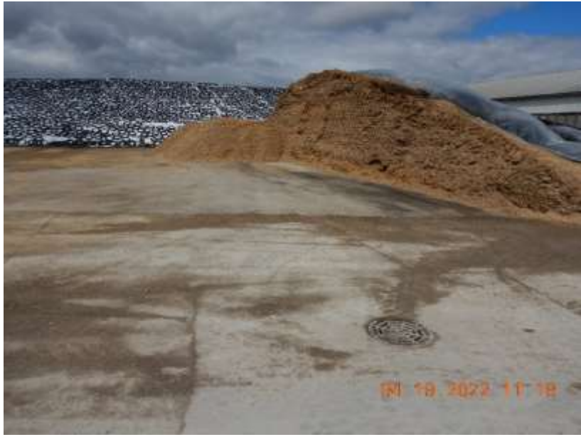
Photo 60. An area where gravel was placed over broken and missing concrete. This photo was taken facing south.
