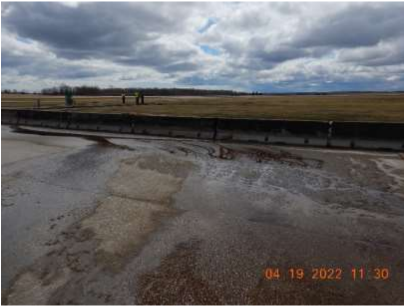
Photo 65. The runoff collection system for the feed storage area at the Main Site. This is located on the southeast corner of the FSA. This photo was taken facing south.
