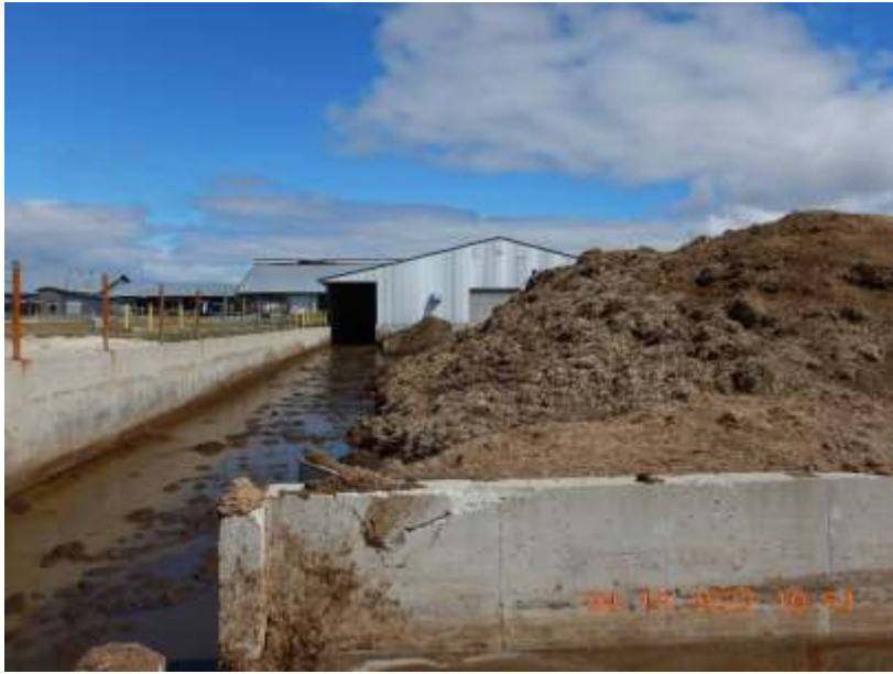
Photo 15. The solid manure storage area located adjacent to the sand lane. Runoff gravity flows into the sand lane. This photo was taken facing northeast.
