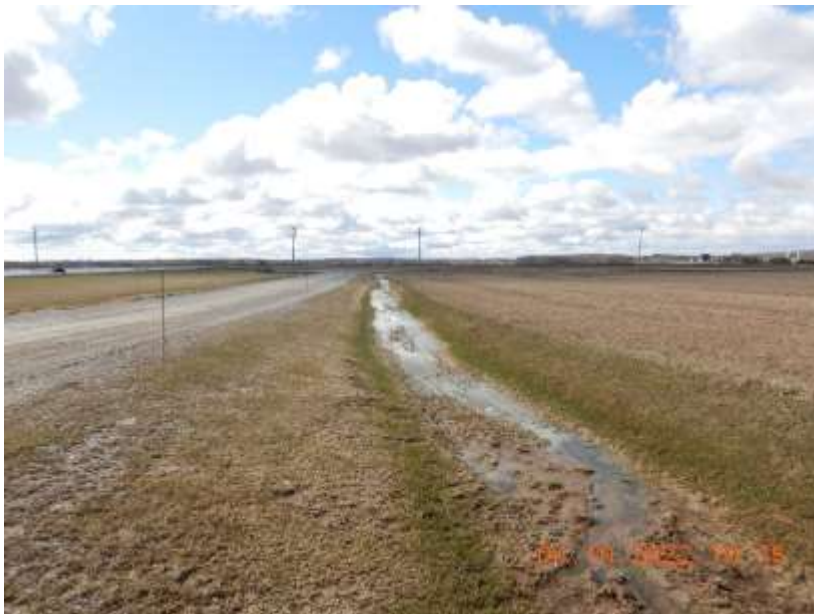
Photo 100. A grassed drainage ditch that conveys stormwater south off the production site. This photo was taken facing south.
