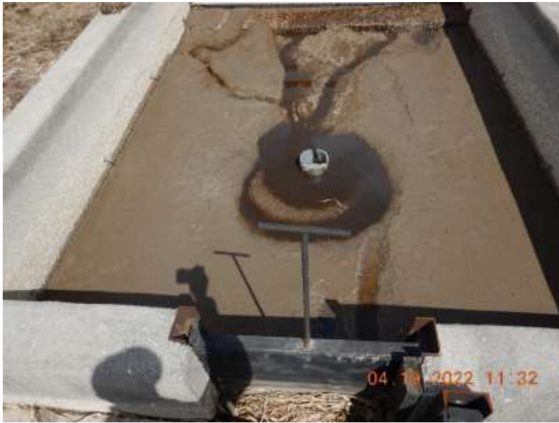
Photo 68. The concrete spreader bar that evenly distributes runoff cross the west vegetated treatment area. This photo was taken facing west.
