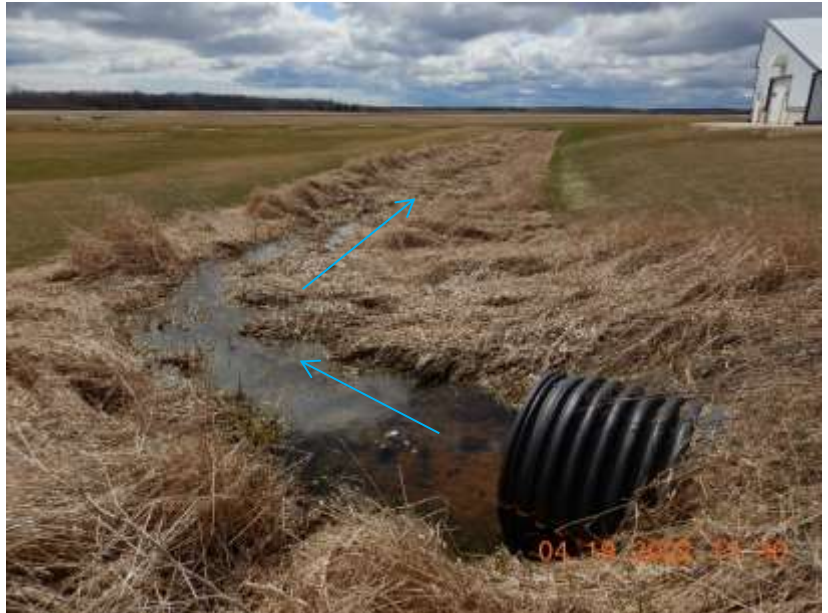
Photo 106. A grassed swale located west of the west VTA that conveys stormwater off the production site.
