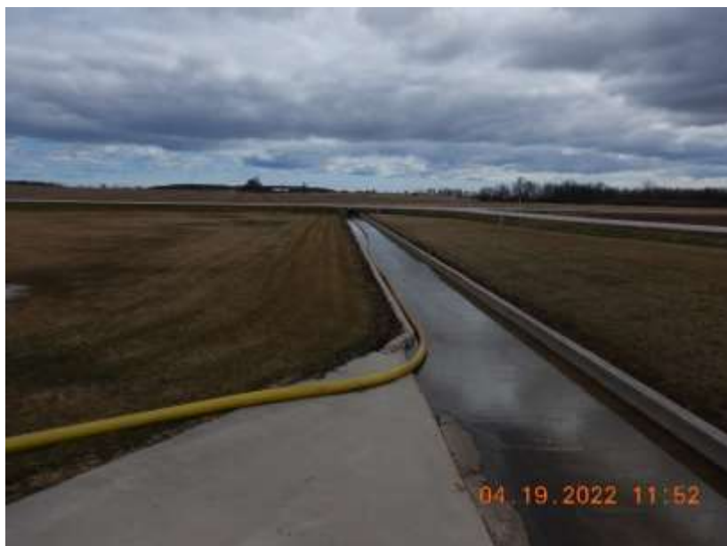
Photo 87. The concrete channel on the south side of the east vegetated treatment area. This channel conveys stormwater off the production site.
