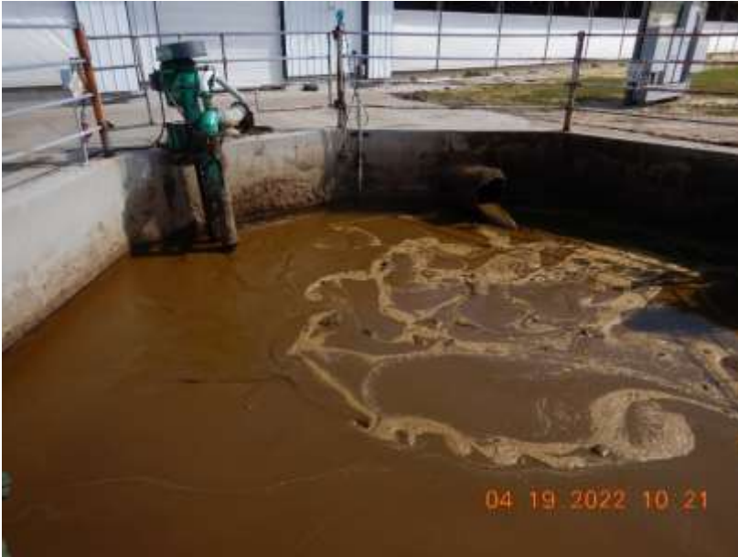
Photo 10. The outlet that discharges manure generated at the Main Site to the north side of the sand lane.
