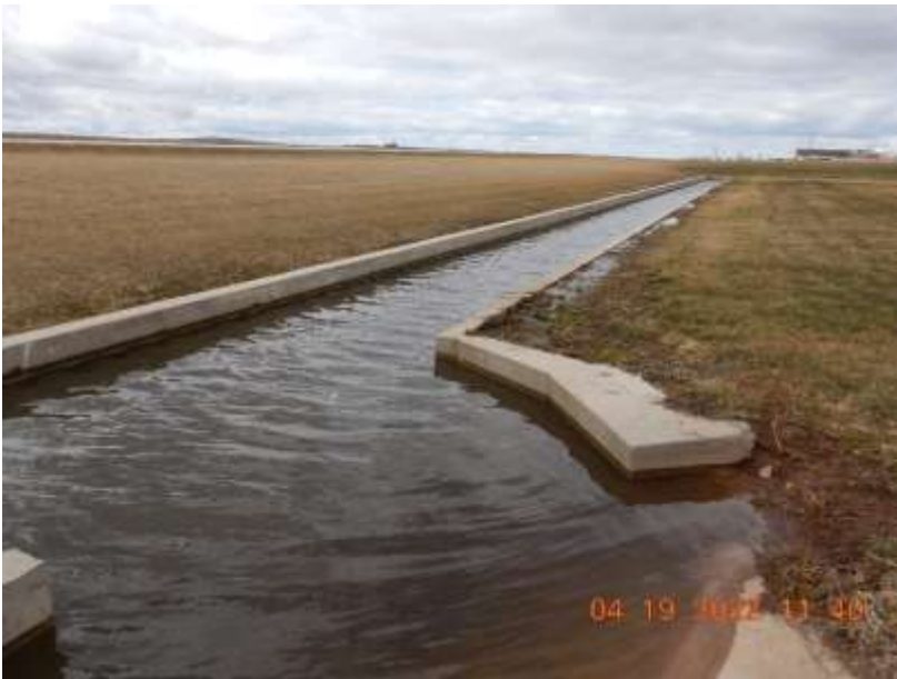
Photo 77. The collection basin for the concrete swale. Runoff can be manually pumped to either the spreader bar or WSF 4 from this location. Stormwater can also flow through the culvert.
