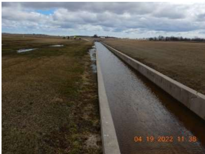
Photo 75. The concrete swale on the south side of the west VTA. The swale conveys stormwater as well as captures runoff that leaves the treatment area. This photo was taken facing east.
