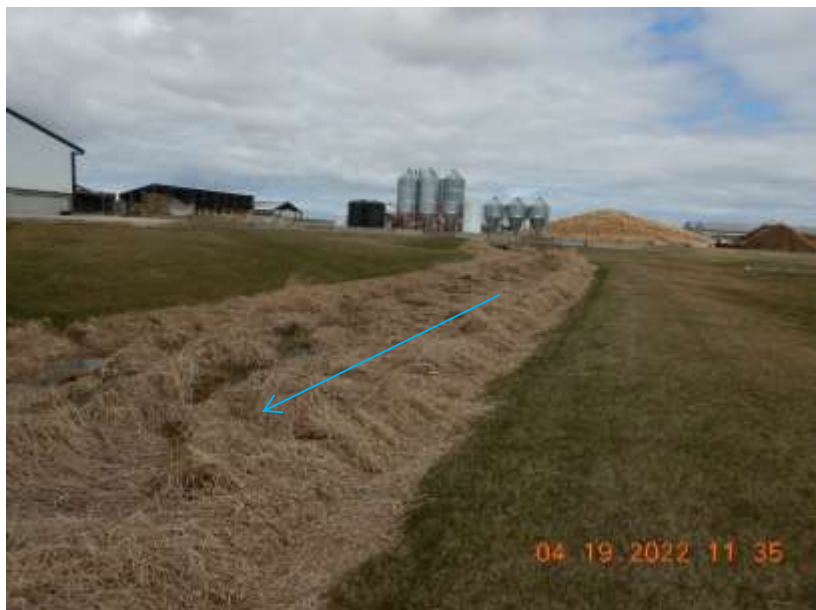
Photo 106. A grassed swale located west of the west VTA that conveys stormwater off the production site.
