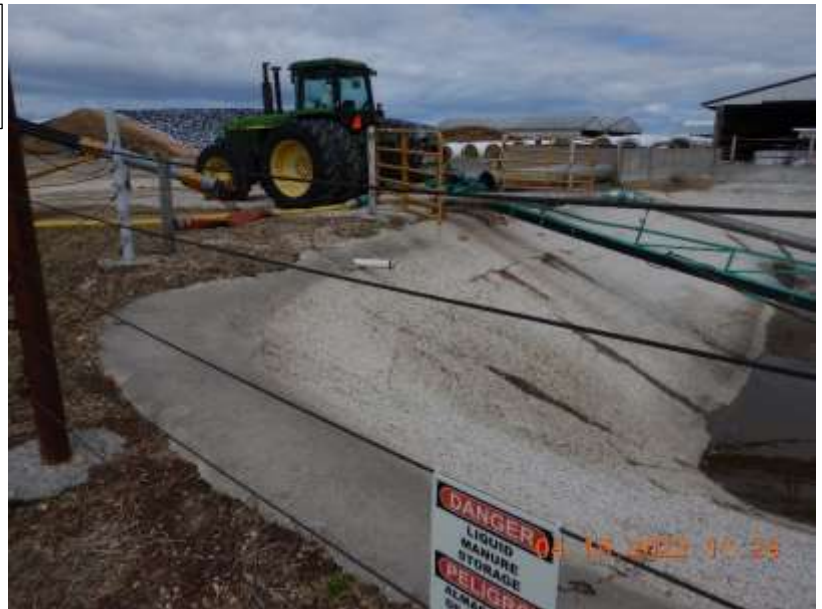
Photo 22. The overland transfer hose that is used to transfer process wastewater from WSF 4 to WSF 3. This photo was taken facing south.
