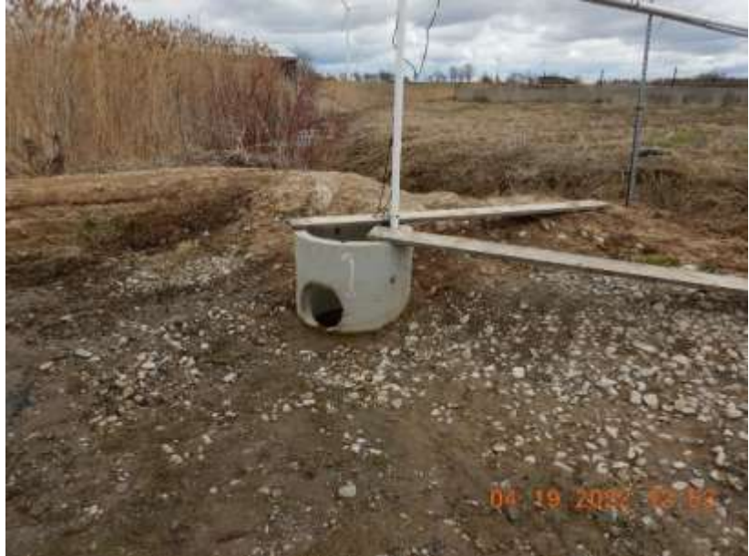
Photo 96. The transfer pipe that conveys runoff from the collection basin to the liquid waste storage facility at the Heifer Dreams site.
