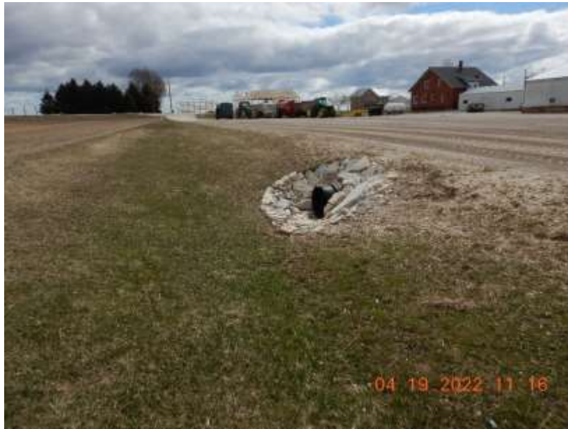
Photo 105. A grassed swale located west of the west VTA that conveys stormwater off the production site.
