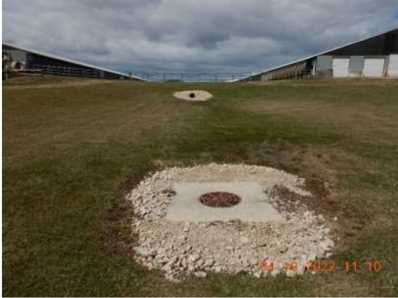
Photo 103. A stormwater culvert that conveys stormwater from the north side of the production site through the site.
