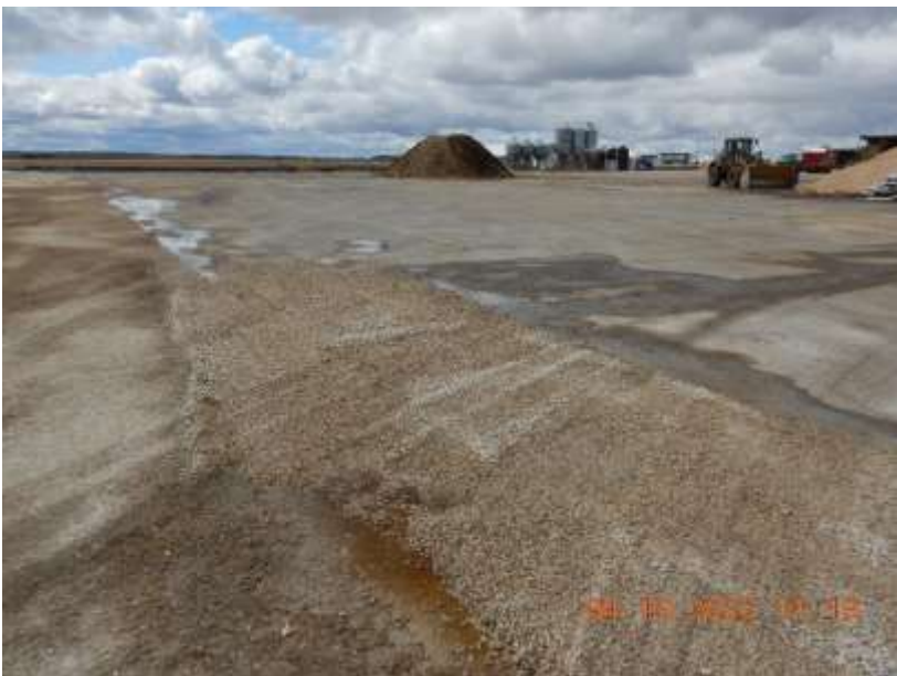
Photo 60. An area where gravel was placed over broken and missing concrete. This photo was taken facing south.
