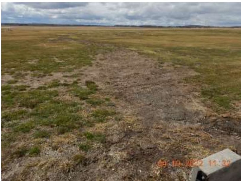
Photo 69. A concentrated flow channel on the east side of the west vegetated treatment area. This photo was taken facing south.
