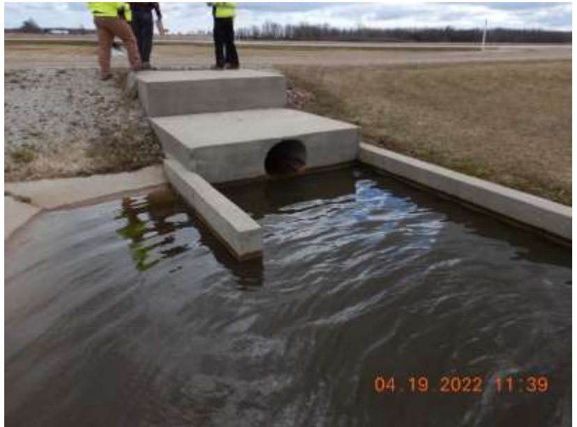
Photo 78. The basin that captures runoff from the concrete swale and pumps the water to either the concrete spreader bar or WSF 4. This photo was taken facing north.
