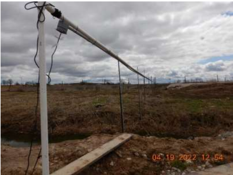
Photo 96. The transfer pipe that conveys runoff from the collection basin to the liquid waste storage facility at the Heifer Dreams site.
