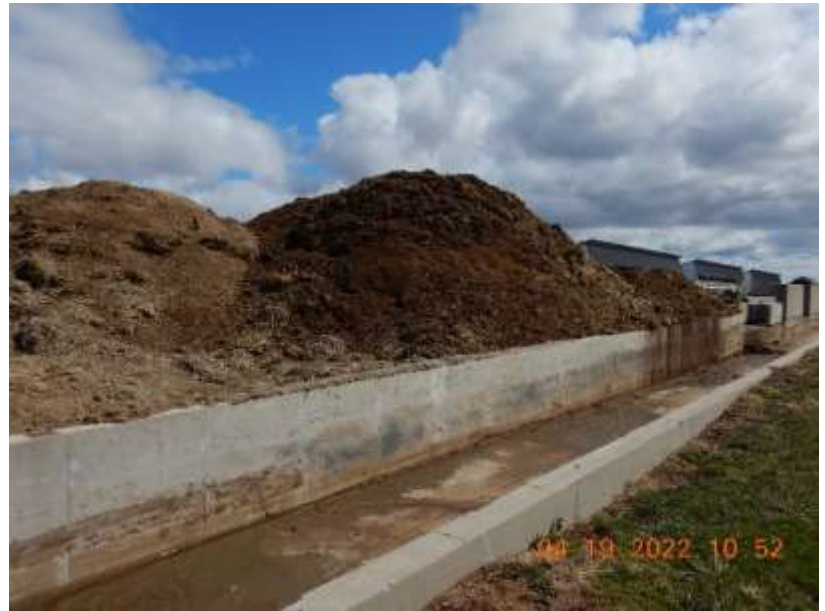
Photo 16. The solid manure storage area located adjacent to the sand lane. Runoff gravity flows into the sand lane. This photo was taken facing north.
