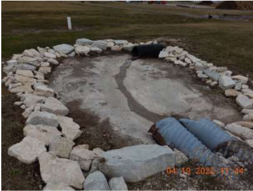
Photo 80. The culverts that convey runoff to the concrete spreader bar for the east VTA, seen in the background. This photo was taken facing east.
