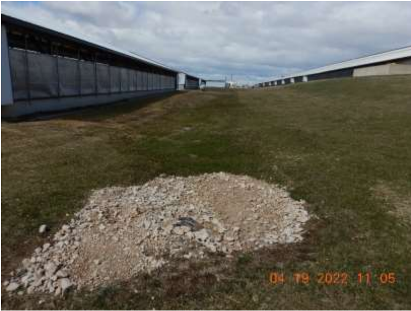
Photo 102. A stormwater surface inlet that accepts conveys stormwater from the grassed swale between barns.
