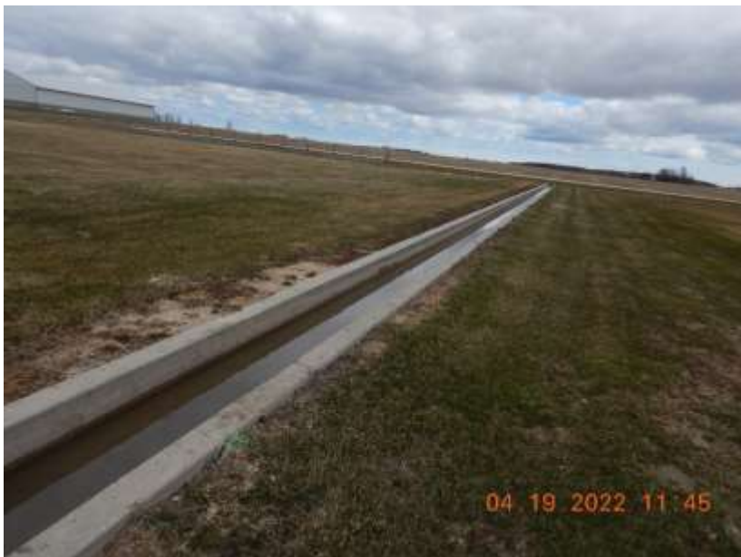
Photo 81. The concrete spreader bar for the east vegetated treatment area.
