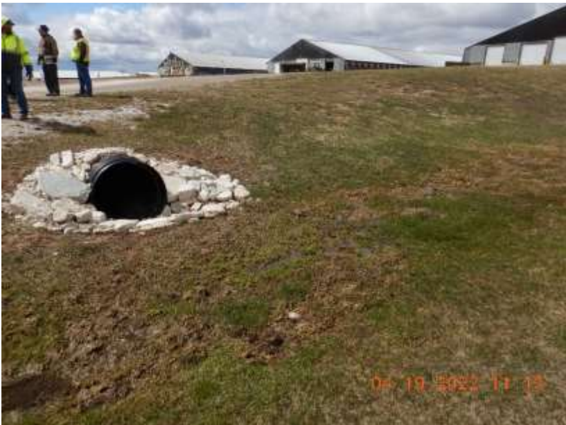
Photo 103. A stormwater culvert that conveys stormwater from the north side of the production site through the site.
