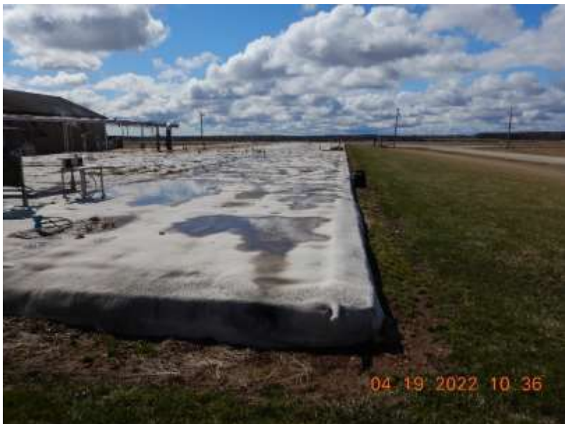
Photo 49. The anaerobic digester located west of the solid separation building. All manure generated at Main Site is digested prior to being transferred to permanent storage.
