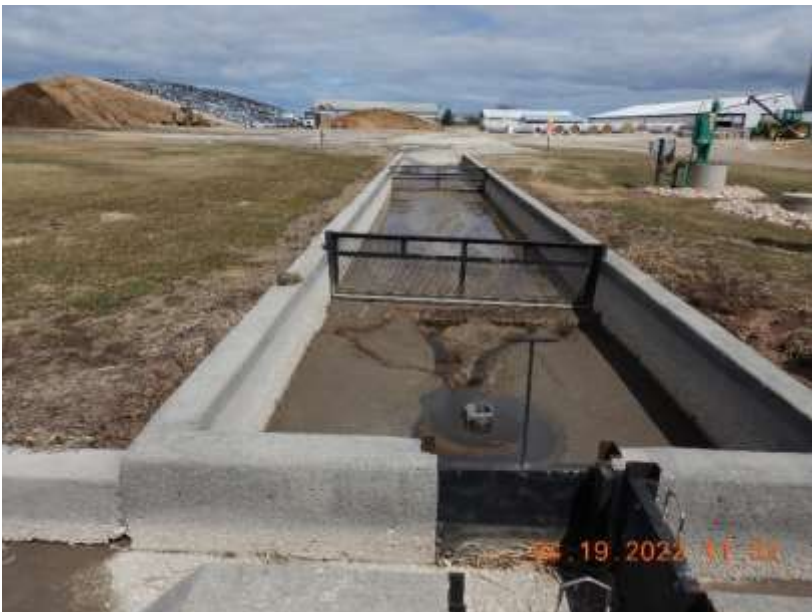
Photo 66. The runoff collection system for the feed storage area at the Main Site. This is located on the southeast corner of the FSA. This photo was taken facing north.
