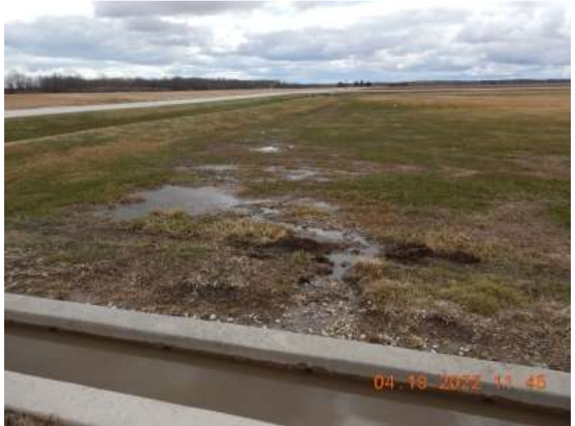
Photo 84. A concentrated flow channel coming from the east side of the concrete spreader bar for the east VTA. This photo was taken facing west.
