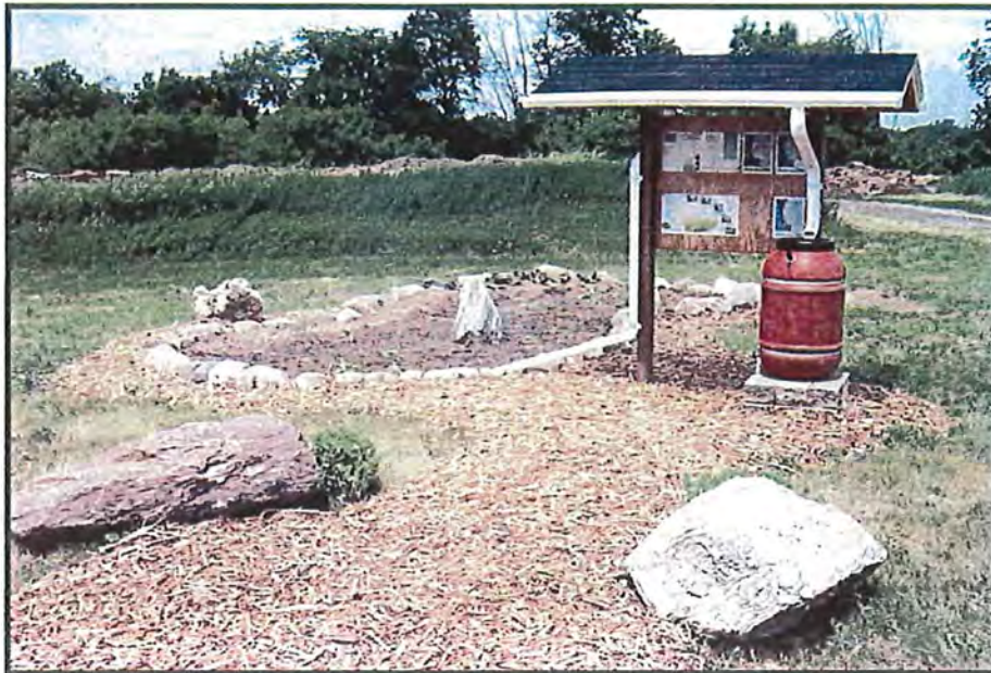
Rain Garden - finished view. Rain barrels can be purchased through MMSD
