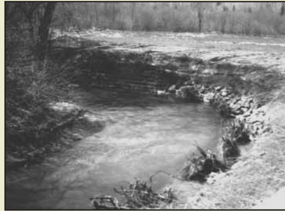
Streambank stabilization within the Whittlesey Creek Watershed.
